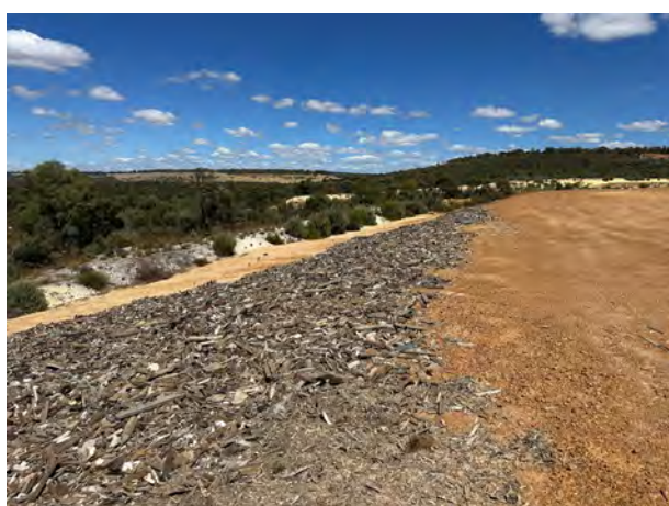
Figure 2: Wood mulch placed to ameliorate erosion around Cell 1
