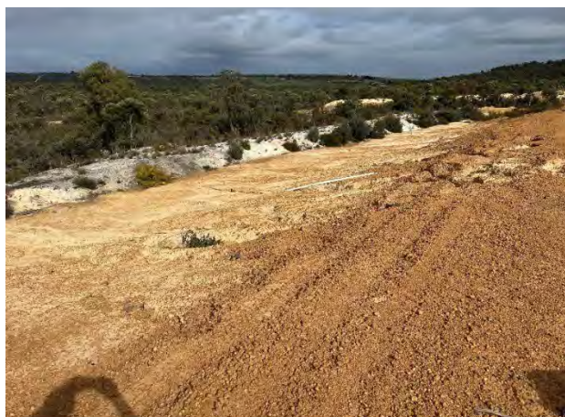
Figure 1: Erosion observed around Cell 1
